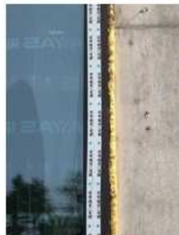
缝隙用发泡胶填塞密封
